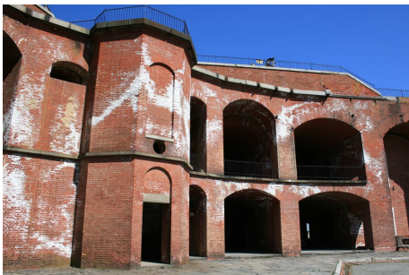
Circular stairway near northeast bastion
