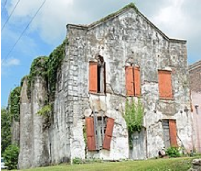
Building at Broad and Screven, the only existing building that survived the 1863 burning of Darien by the US Army
